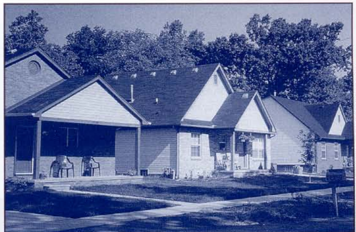
New homes were constructed in this Brownstown Charter Township subdivision as a result of infrastructure improvements funded by a DDA.
