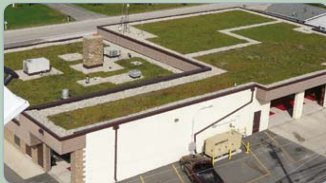
Ira Township's (St. Clair Co.) 'green roof'
